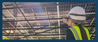
A 346 kW carport at Mount Rushmore both protects cars from the weather and provides electricity for the park. The carport is estimated to save the park over \$40,000 annually with its low cost electricity.
