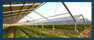
New Mexico State is studying the impacts of co-locating solar panels and chiles. This practice, called agrivoltaics, could reduce heat stress on the crops while also helping farmers generate electricity for operations.
