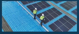
Lyman Products added a 698.87 kW rooftop array that will generate 739 MWh of clean energy each year. This will save the Connecticut manufacturer \$328,000 over the array's lifespan.
