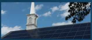
Watauga Avenue Presbyterian Church added 41 rooftop solar panels that will generate around 66,000 kWh of low cost electricity annually. This will supply 40% of the electricity for the church.
