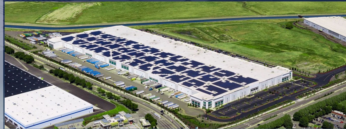
Amazon Distribution Center | Tracy, CA | Photo Courtesy of EnterSolar
