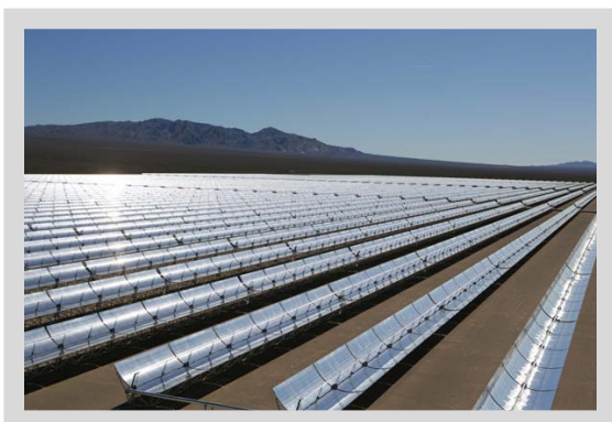
The 64 MW Nevada Solar One parabolic trough facility in Boulder City, Nev., was completed in June 2007.
